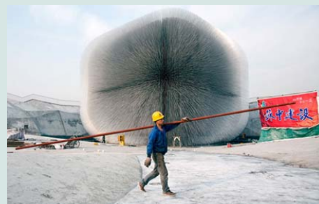
The UK Pavilion known as the "Seed Cathedral". Its wooden structure is pierced by more than 60,000 acrylic rods containing a variety of seeds from different plants.
